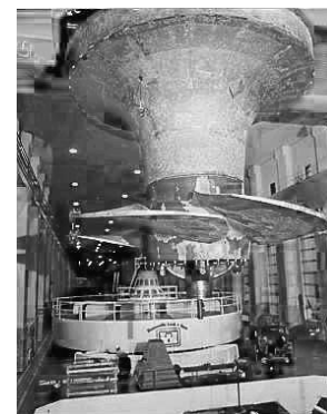
Kaplan Turbine at Bonneville Dam after 61 years in service
